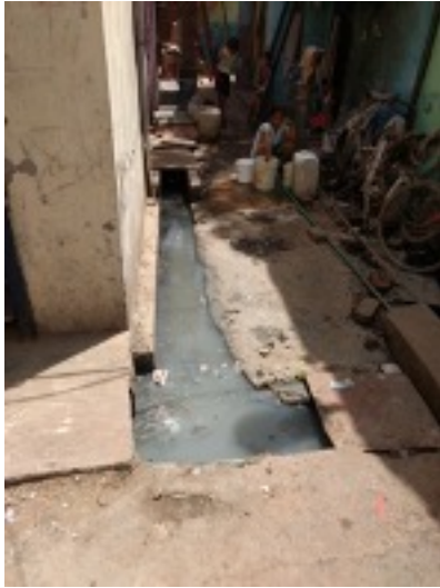
(a) Internal drains run next to houses, often close to sources of water supply, thus contaminating drinking water.
